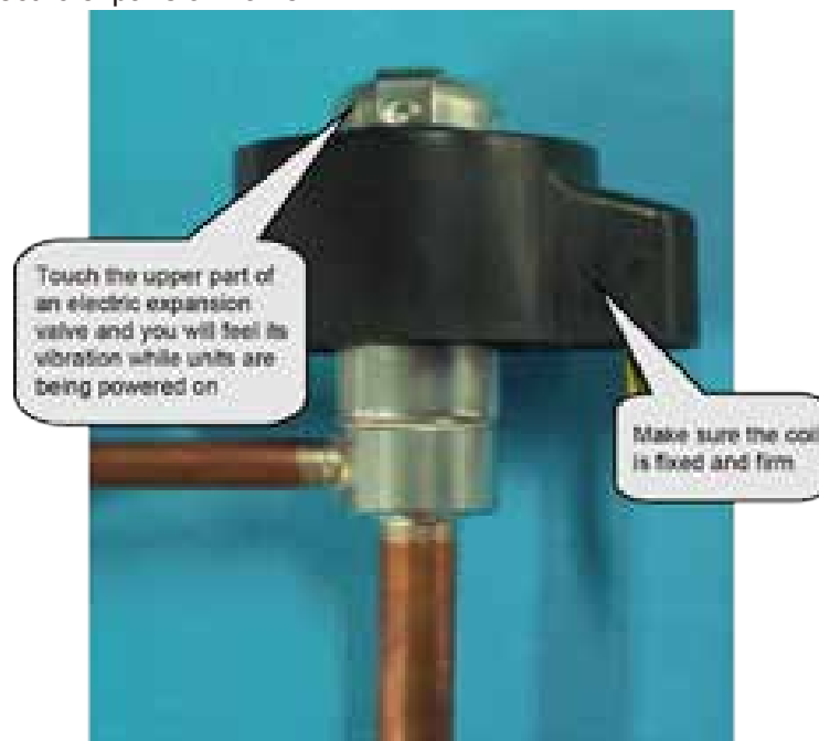
Description of electric expansion valve:
